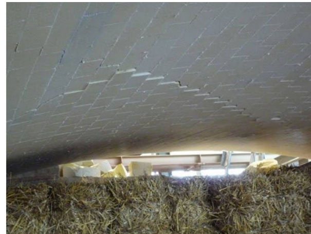
Wrong choice of refractory material
