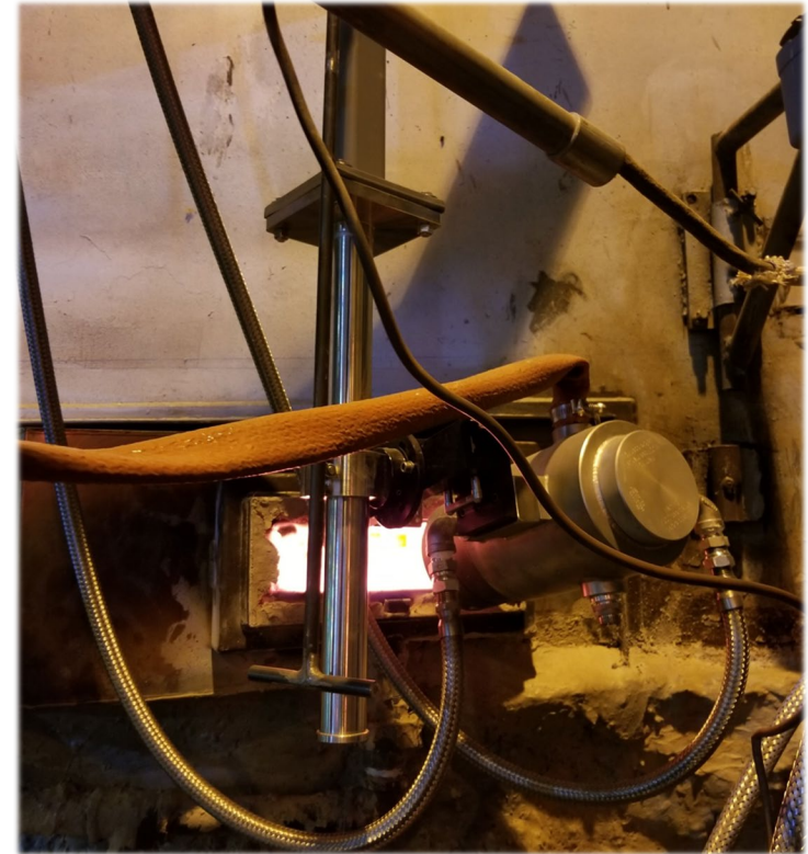
Camera installation at float bath corner view windows
