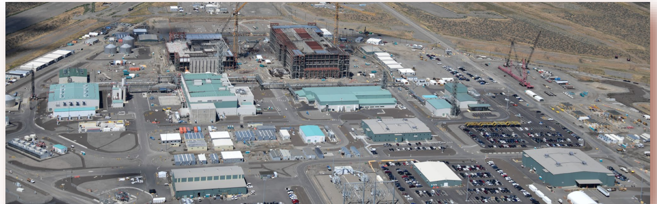
Waste Treatment and Immobilization Plant (WTP)
